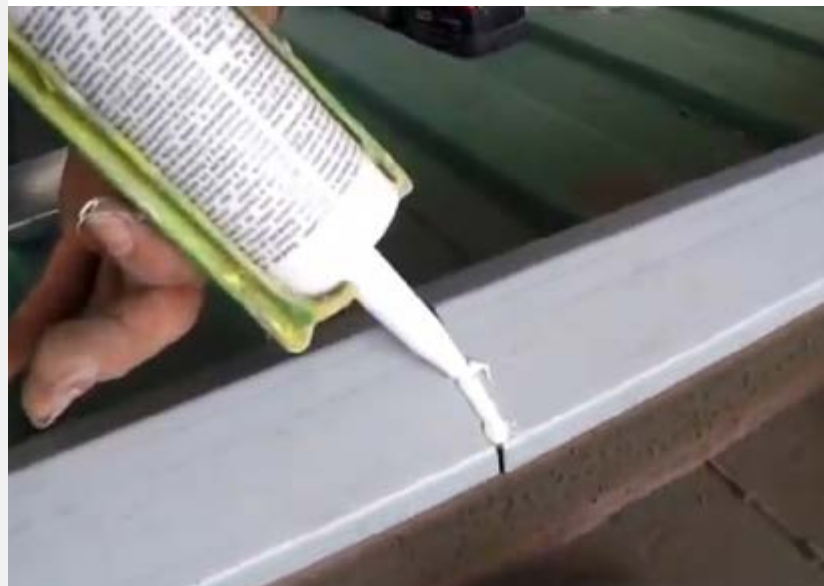
Above: Caulking seals the seam between roof top ridge caps
