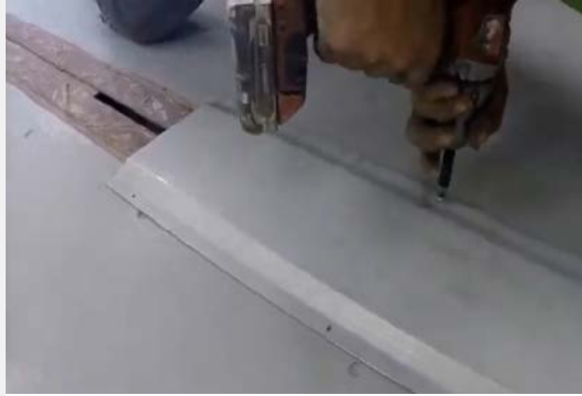
Above: Interior threshold to interior floor
