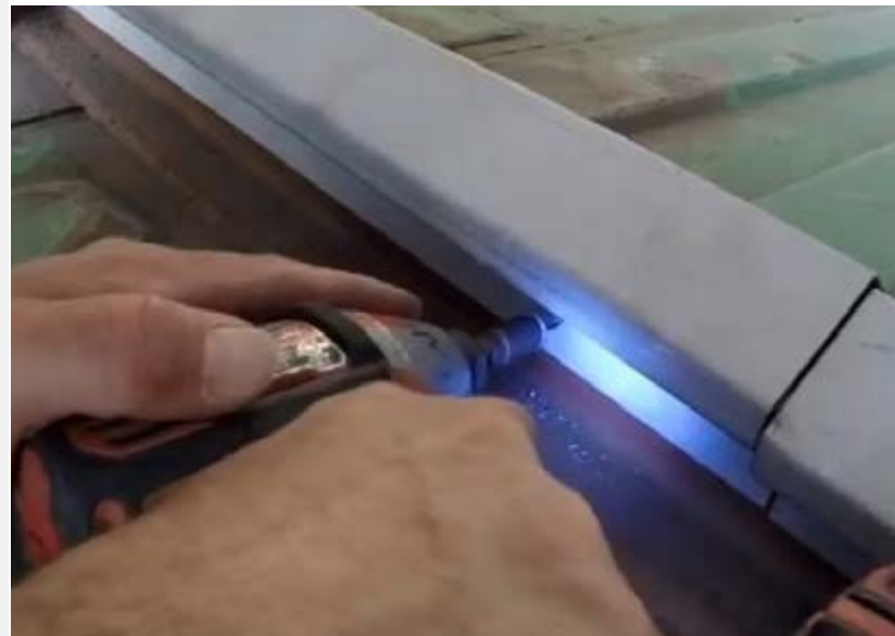
Above: Ridge cap that covers the seam between container roofs drilled into place
